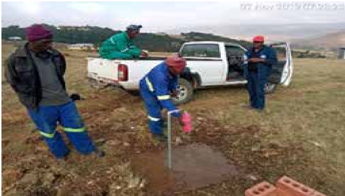
Construction of Spring Water Protection – Qwidlana Village in Mzimvubu LM
